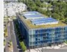
Green roofs absorb rain, enhance insulation, and support local biodiversity, making them an eco-friendly, cost-effective, and low-maintenance complement to rainwater systems for sustainable buildings. When combined with solar PV installations, they further reduce the local GHG emission footprint, maximizing environmental benefits.
