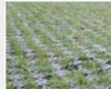
Perfo-AK tiles create a permeable parking surface by being compacted into a gravel layer with a prepared sub-base. This design allows rainwater to seep into the ground, reducing surface runoff, mitigating temperature risks, and supporting healthier vegetation. Additionally, it helps combat urban heat island effects through natural cooling and enhances resilience to heatwaves and drought by promoting groundwater recharge.
